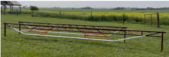
Completed 20 foot span bridge.
