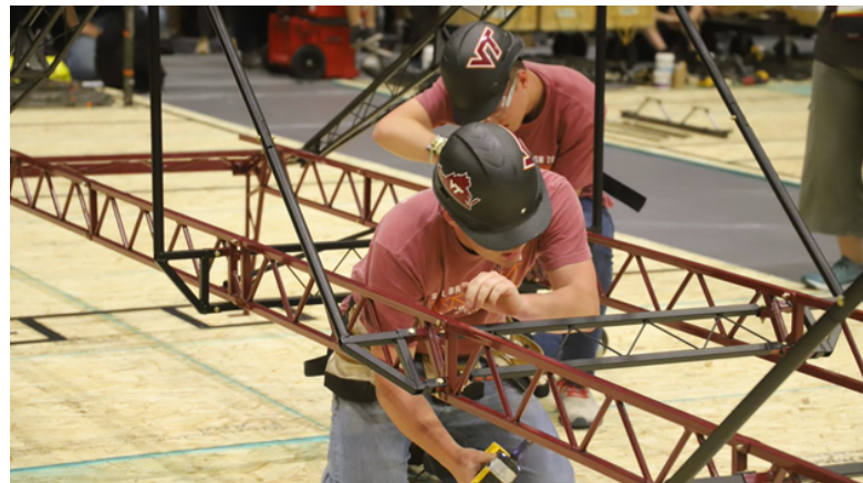
SBT member during the timed construction event in San Diego, California.
